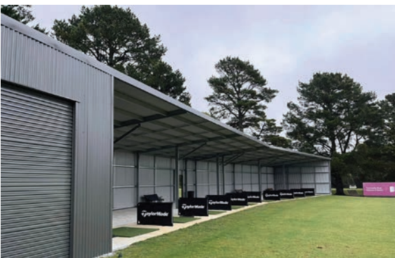
Gisborne Golf Club's driving range shelter is completed, December 2024.
