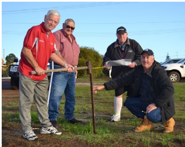
Community Bank Collie directors Ian Miffing, John Piavanini, Ken Smallwood and 101.3FM building project manager Mark Sanders banging in the first marker of the new building.
